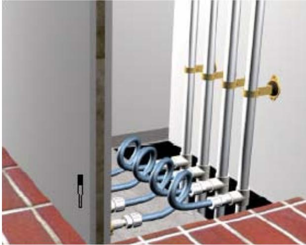
Figura CAL-05. Conectores flexibles
